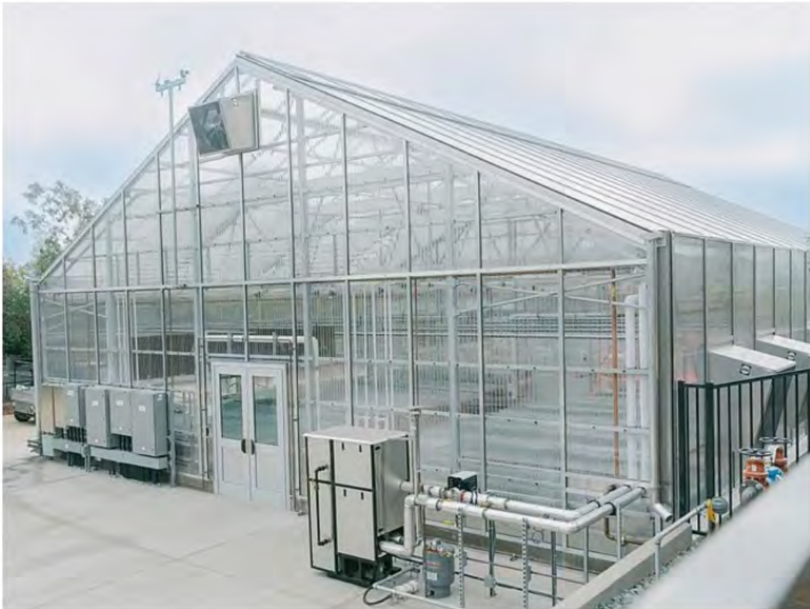
A $19.4 million renovation and expansion of the Cuyamaca College Horticulture Center included a new greenhouse. Photo courtesy of Grossmont-Cuyamaca Community College District.
