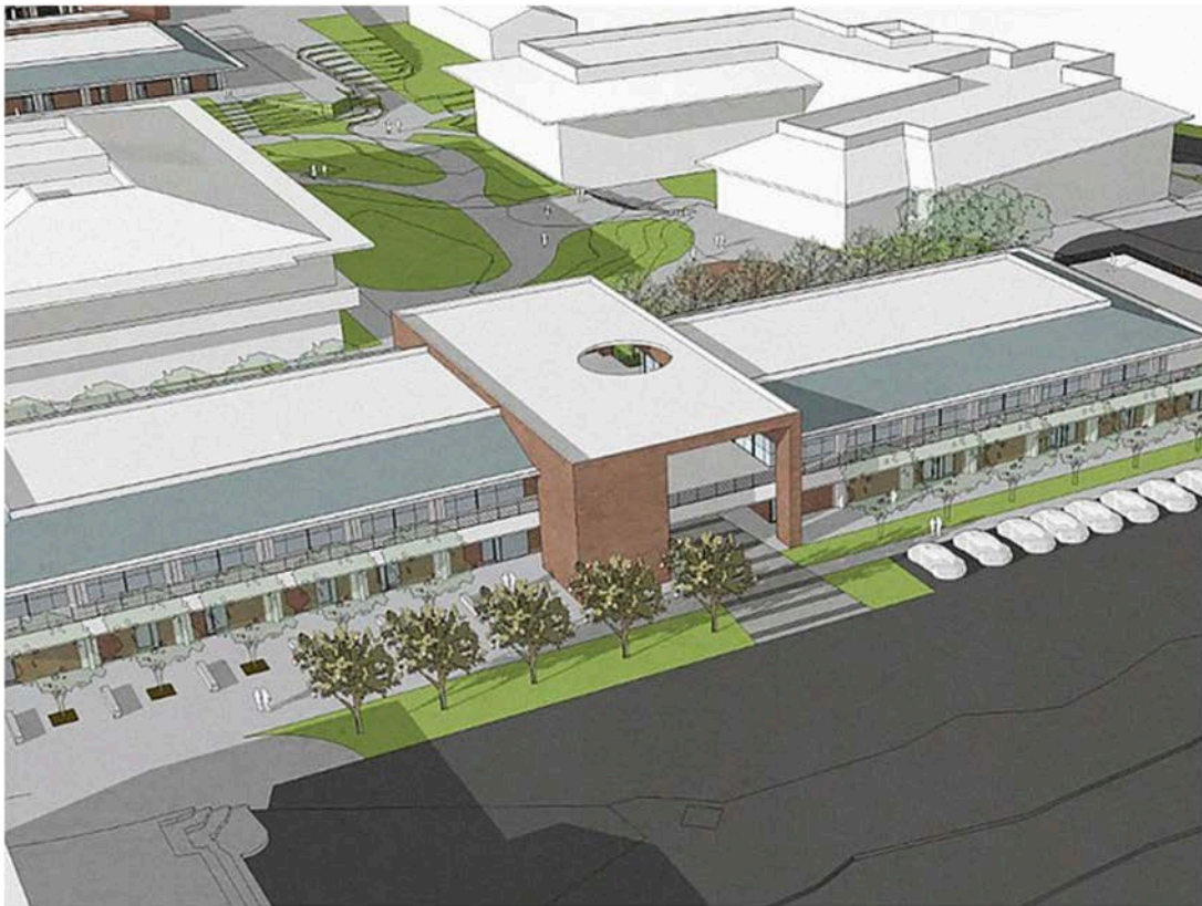
Rendering Courtesy of Gafcon, Inc. A new Science, Math and Career Complex at Grossmont College is scheduled for completion in April 2023.
