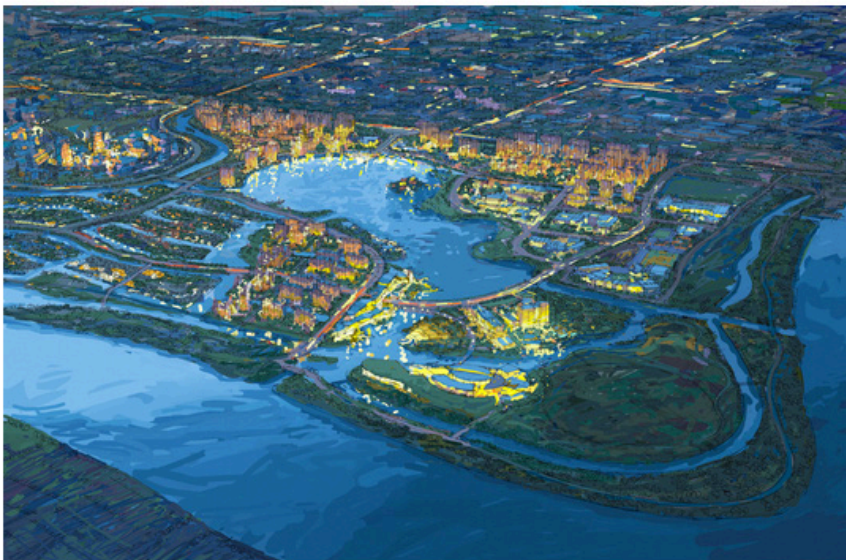
Rendering of the Zizhu Purple Bay residential community. (Courtesy of Gafcon Inc.)
